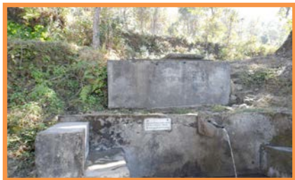
1: Drinking water tap
